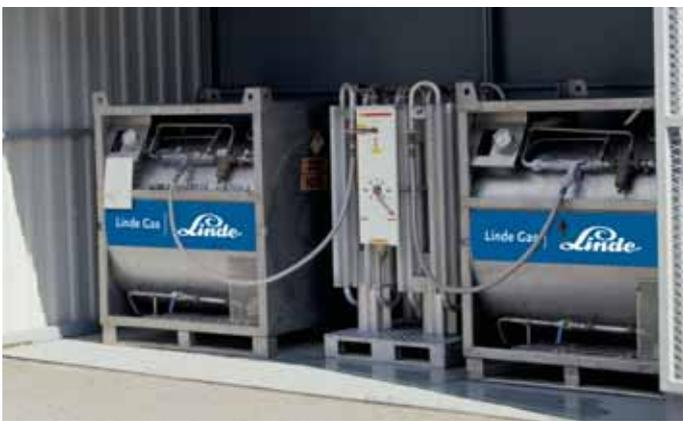
LIN tanks operate on the same principles regardless of the size or amount of LIN they store. The vessel has two walls, an inner shell made from stainless steel to accommodate the cryogenic temperatures and the outer shell constructed of structural steel. The space between the two walls contains an insulating material. Insi-
